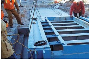
**Advanced Modular Construction** - A single module has a weigh rail length of 12'6" (3.8 m). Two modules give a weigh rail length of 26' (7.92 m). Standard version with exposed rail or flush deck version available.
